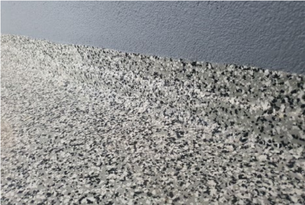
Goondiwindi SHS - Amenties Block Coving and Flake Floor
