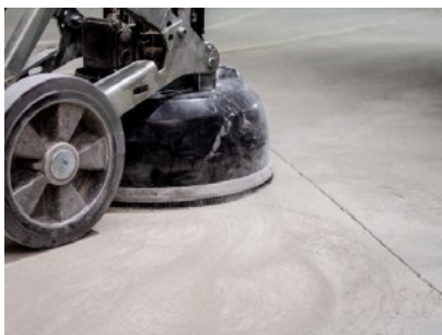
CONCRETE GRINDING
