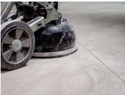
CONCRETE GRINDING
